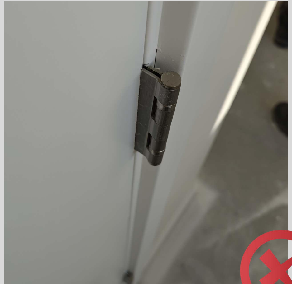
Standard hinge, thickness not suitable, protrudes noticeably
